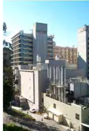
Parnassus Services Building and Central Utility Plant
