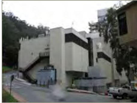
Central Utility Plant
