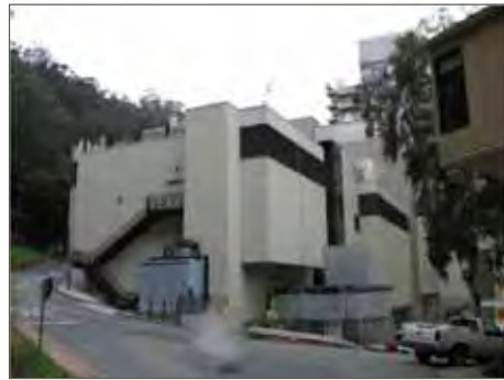
Central Utility Plant
