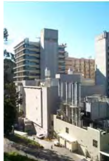
Parnassus Services Building and Central Utility Plant
